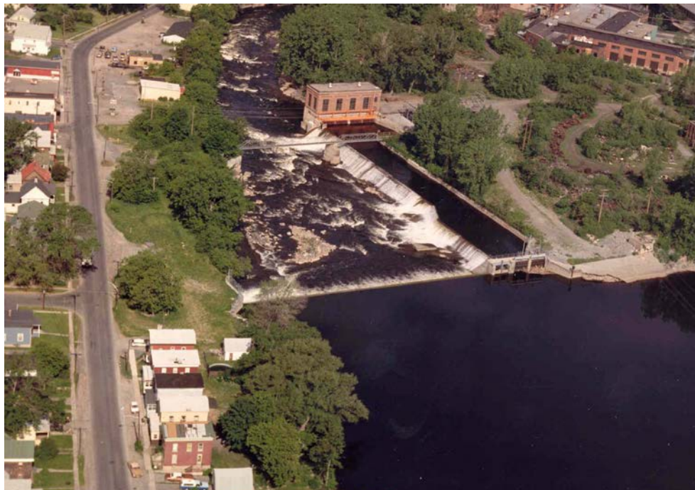
Figure 5 - Downstream view of the Sewalls Development, which is located within the City of Watertown.
