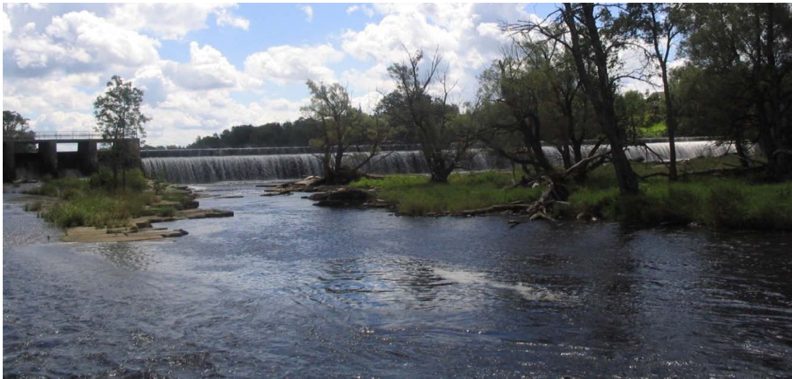
Figure 2 - The Deferiet dam, with 3-foot pneumatic flashboards
