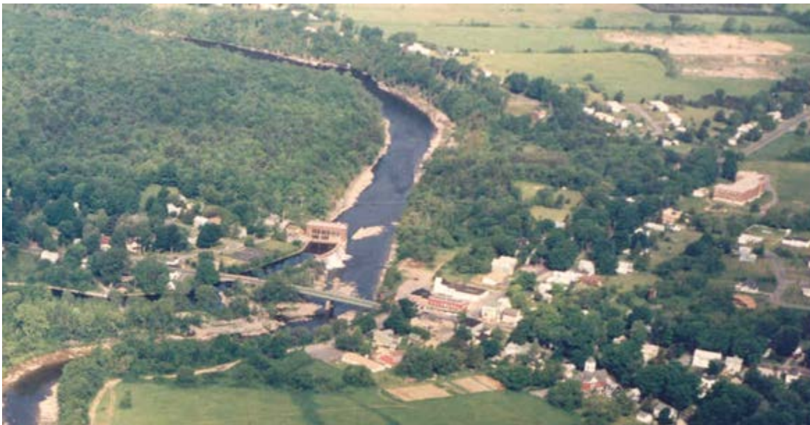
Figure 3 - Downstream view of power canal and bypassed reach at the Kamargo Development
