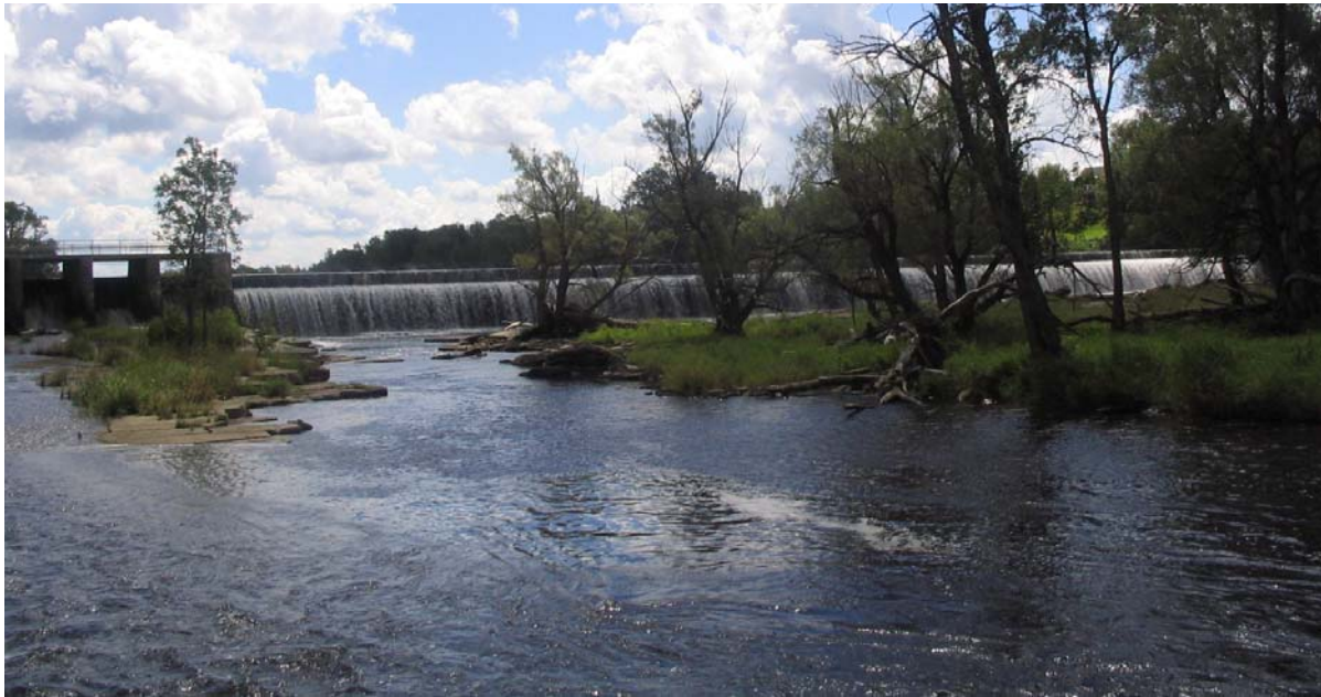
Figure 2. The Deferiet dam, with 3-foot pneumatic flashboards
