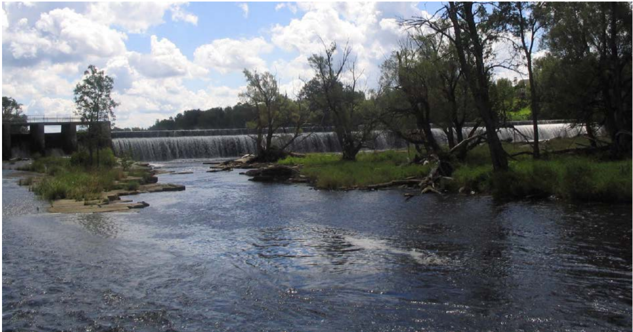
Deferiet dam with 3-foot pneumatic flashboards
