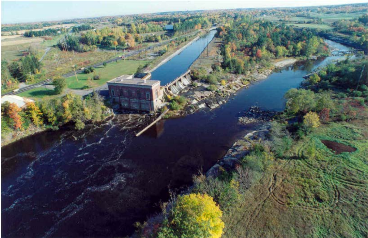
Upstream view of tailrace, powerhouse, canal, and bypassed reach at the Black River Development
