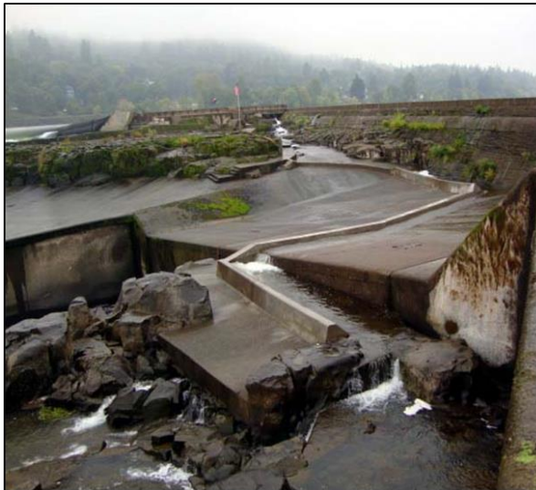
Figure 11. Adult lamprey curb (looking upstream) on top of ODFW Fish Ladder (left). Lamprey exit gate (right).
