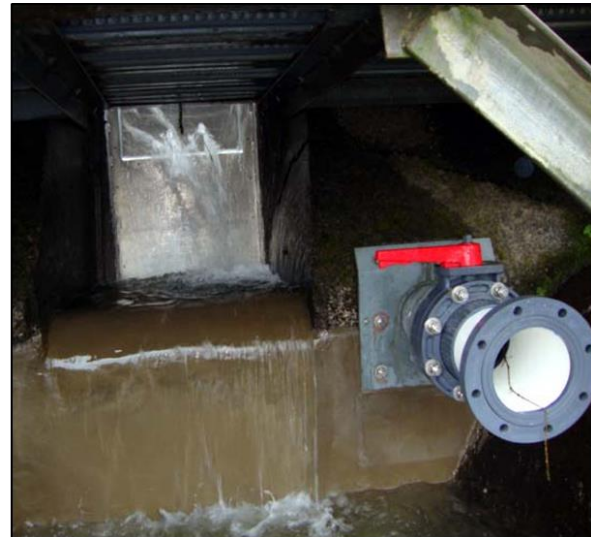
Figure 11. Adult lamprey curb (looking upstream) on top of ODFW Fish Ladder (left). Lamprey exit gate (right).
