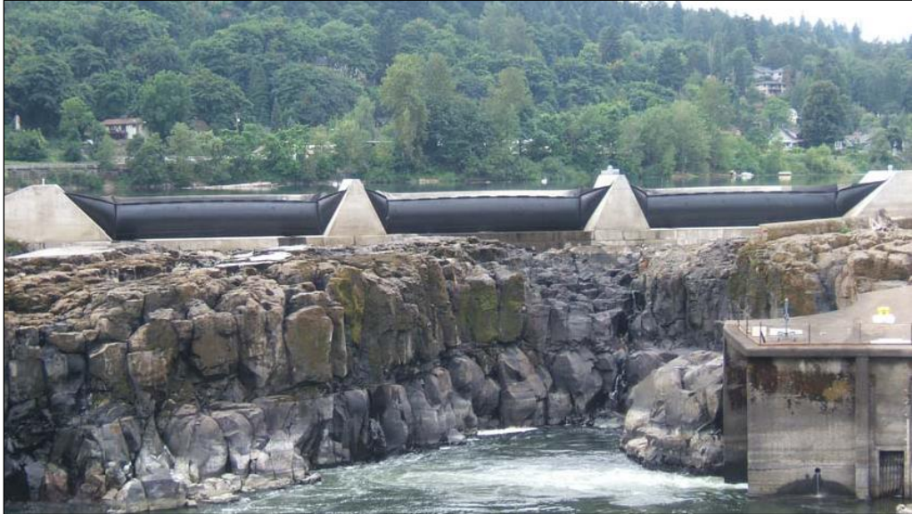
Figure 10. Flow Control Structure at apex of Falls. It consists of three inflatable bladder gates. Picture shows FCS in fully raised (closed) position.
