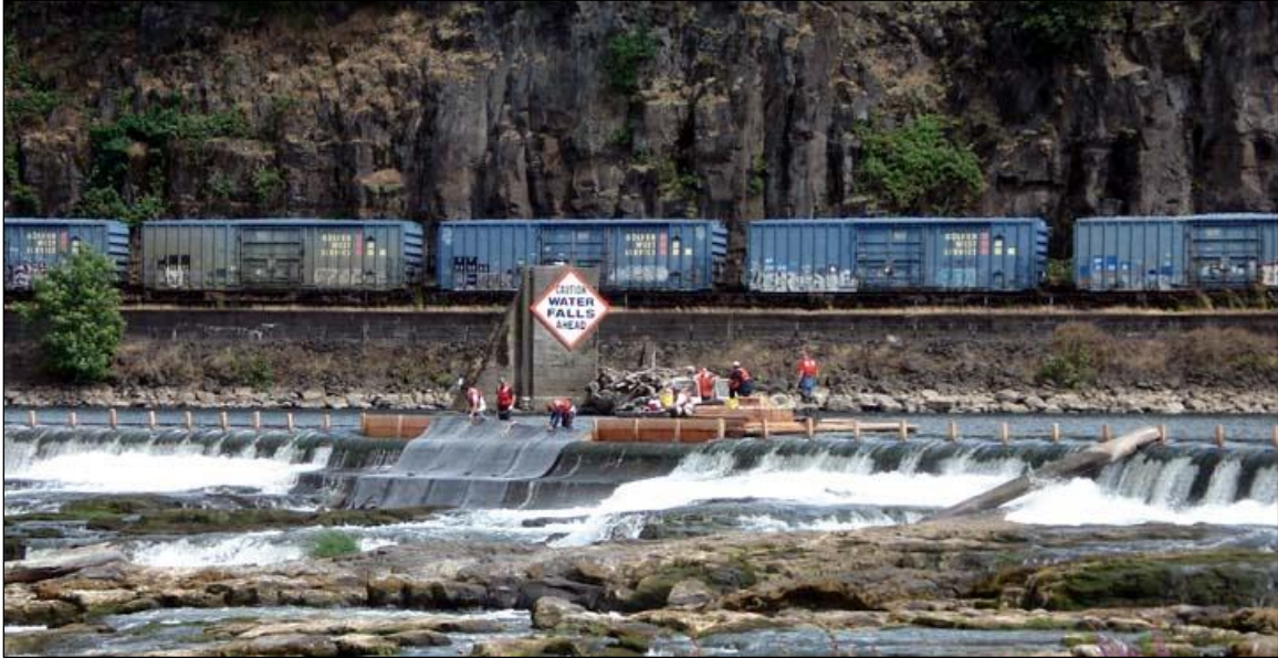
Figure 12. Installation of lamprey passage ramp
