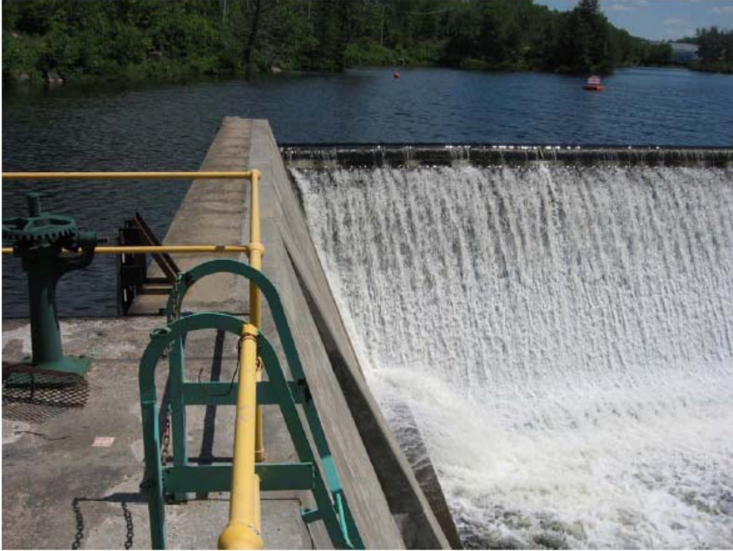
Lower Newton Falls Forebay Wall and Spillway
