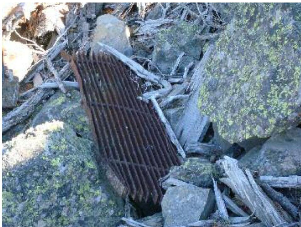
Photo 8: Photo of the discarded trashrack and debris located adjacent to the stairs to the powerhouse that needs to be removed. This is a follow up item.
