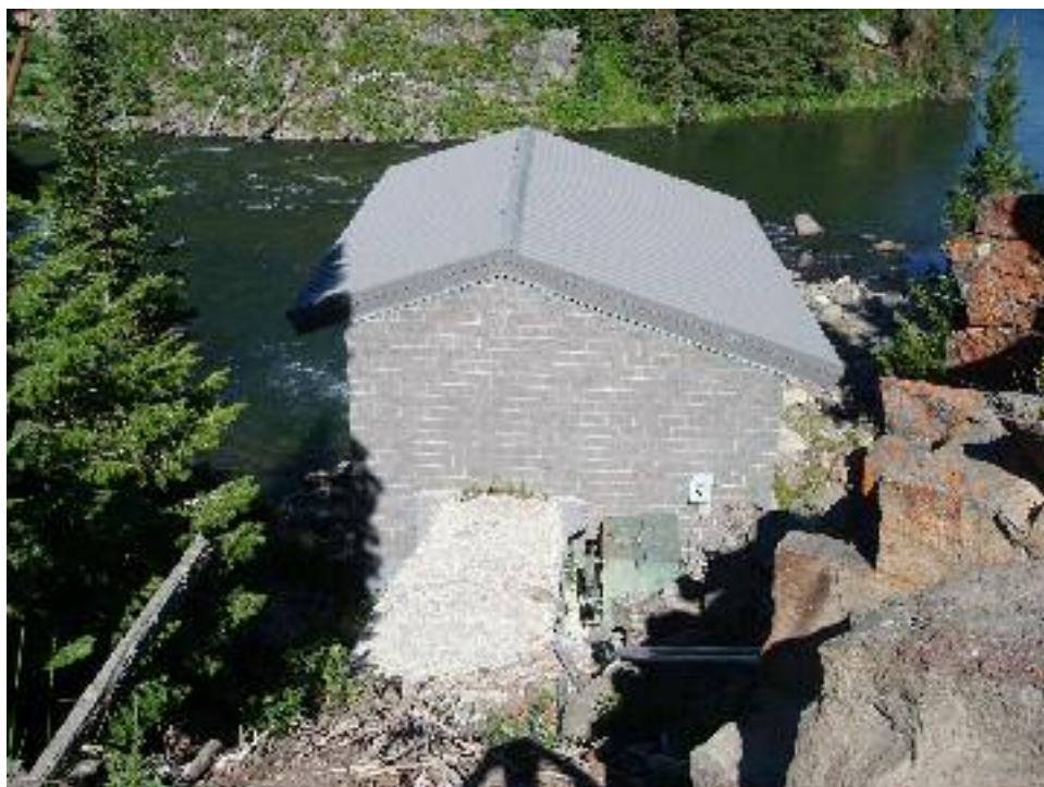
Photo 6: View looking west at the penstock towards the powerhouse. Henry's Fork River is in the background.
