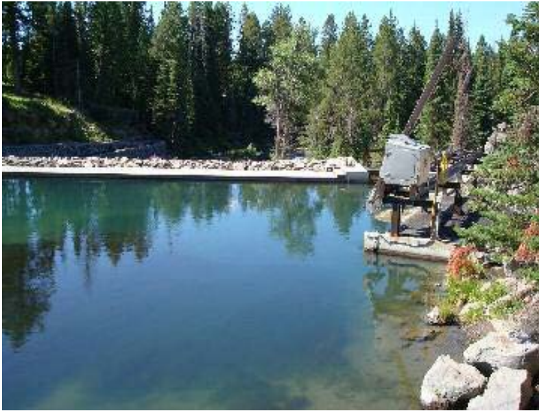
PHOTO 3 DOWNSTREAM VIEW FROM RESERVOIR INCLUDING TRASHRACK AND AUTOMATED RAKE TO RIGHT
