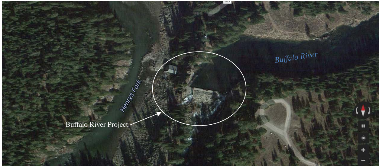
PHOTO 1-1 BUFFALO RIVER HYDROELECTRIC PROJECT
