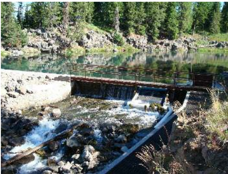
PHOTO 4 UPSTREAM VIEW OF SPILLWAY INCLUDING THE PROJECT FISHWAY (RIGHT)
