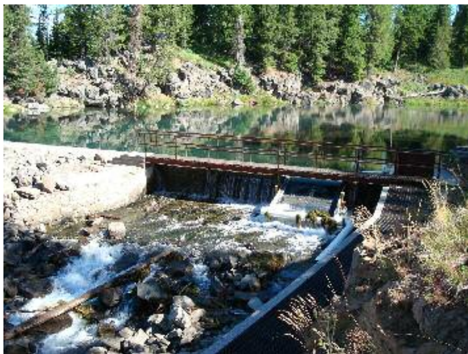
Photo 2: View looking north from downstream showing the spillway. The fishway is located along the right shoreline.
