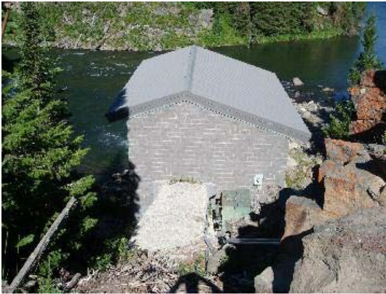
PHOTO 6 PROJECT PENSTOCK AND POWERHOUSE
