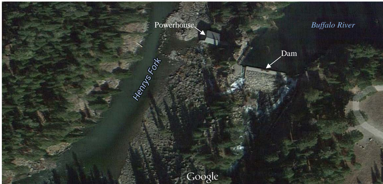
PHOTO 1 BUFFALO RIVER HYDROELECTRIC PROJECT OVERVIEW
