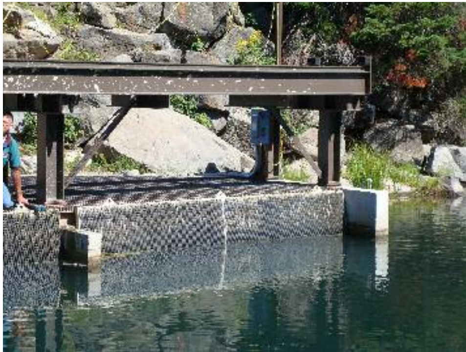
Photo 3: View looking north at the cleaned section of the intake trashrack.
