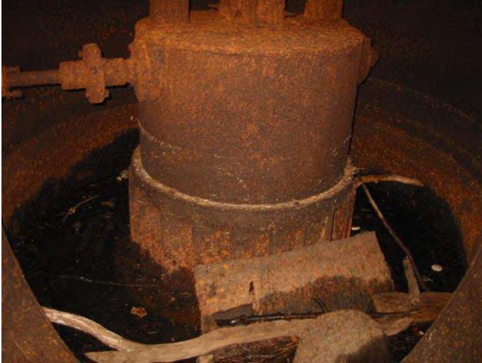
Photo 3 Turbine Within Pressure Case
