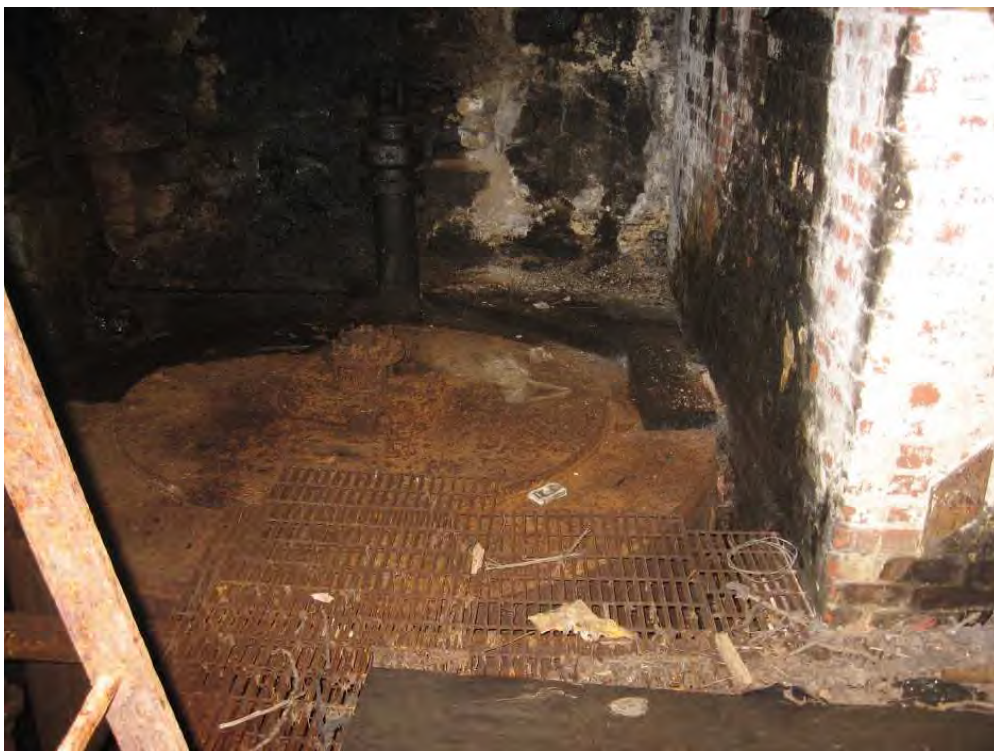
Photo 1. Top of Pressure Casing for Turbine No. 1
