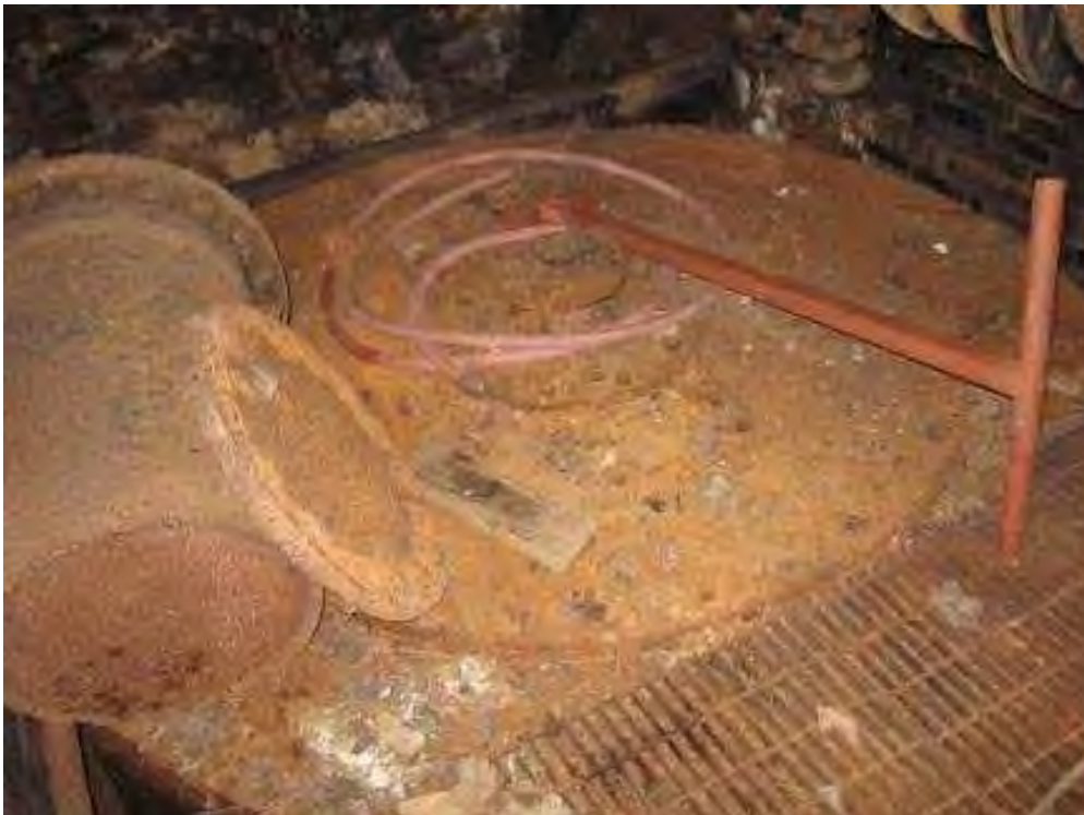
Photo 2. Top of Pressure Casing for Turbine No. 2
