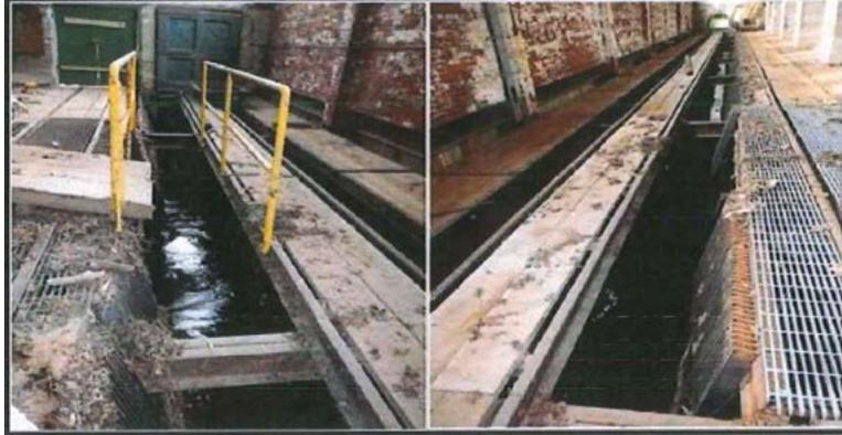
**Figure 8 – Surface Bypasses on West Side (left) and Center of Powerhouse (right).**
