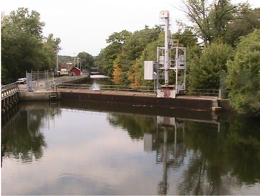
Figure 7. View down canal from gatehouse showing angled trashrack.
