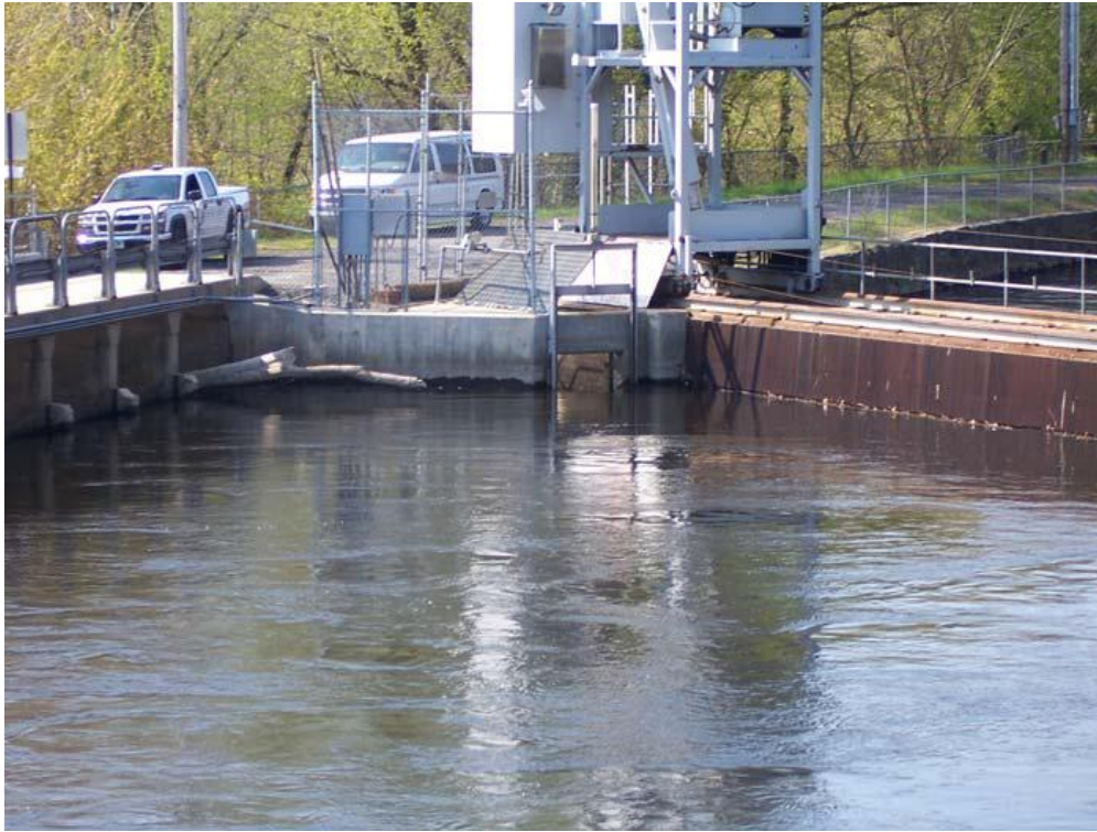
Figure 11. Entrance to downstream passage sluice, angled rack to right.
