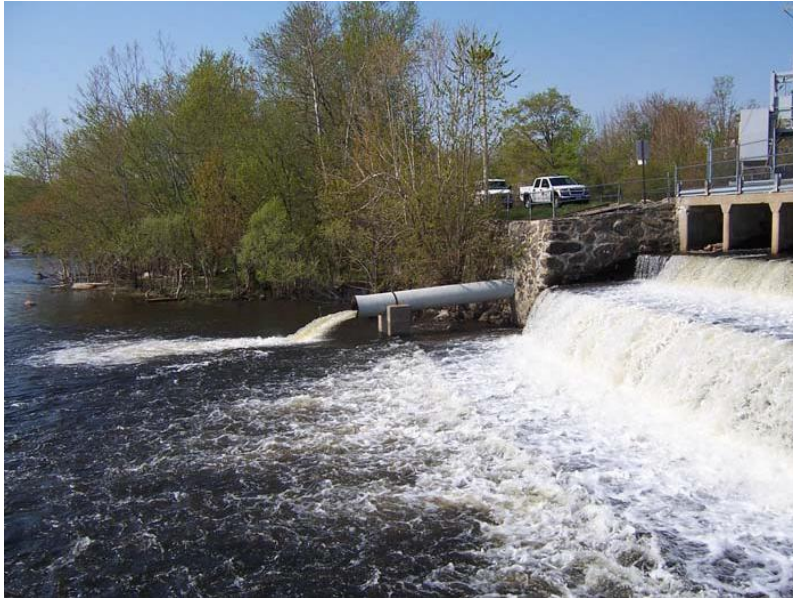
Figure 12. Downstream migrant sluice pipe (36-inch diameter).
