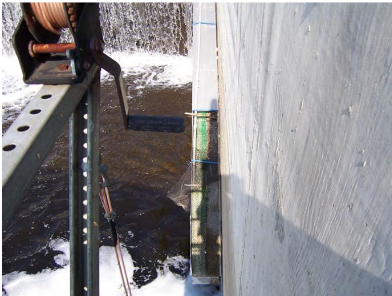
Figure 13. Eel ladder viewed from fish lift structure.
