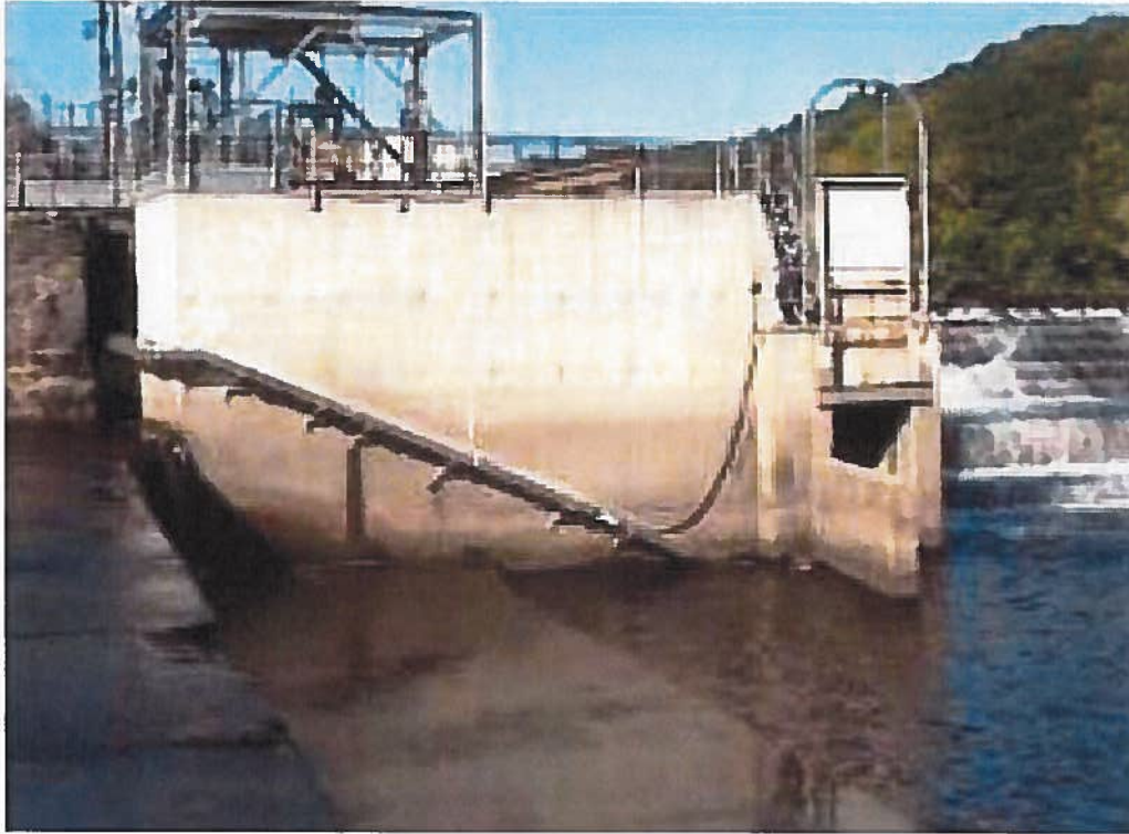
Photo 12C: Upstream Fish Elevator and Eel Ladder
