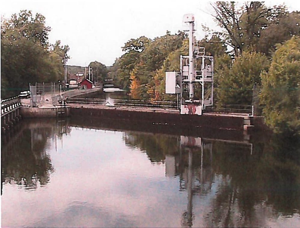
Photo 12D: Canal Angled Bar Rack and Downstream Fish Bypass Inlet
