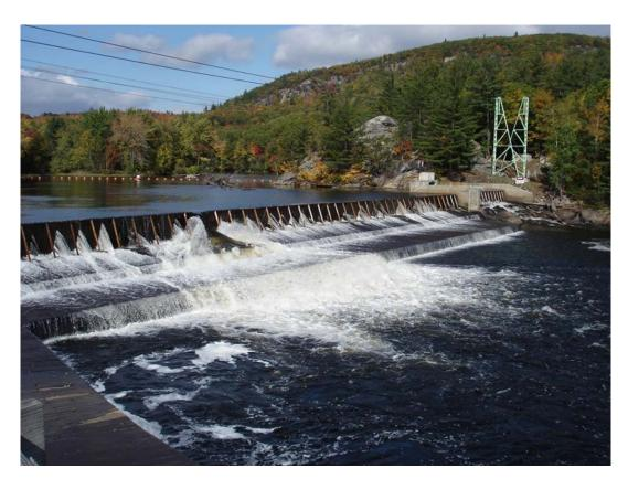
PHOTO 8 VIEW OF LOWERED FLASHBOARD TO PROVIDE MINIMUM FLOW
