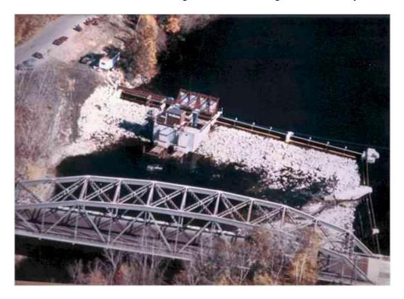
Bulb turbines located in dam with 3 sections of hinged flashboards
