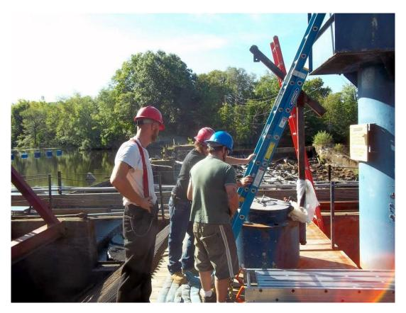
Preparing to remove the bulb top so the gearbox can be extracted from the nose cone.
