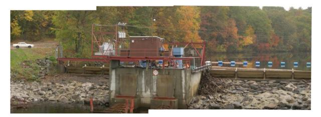
The hydraulic operators lift the hinged flashboards to 4 feet, but could be replaced with inflated runner crest gates
