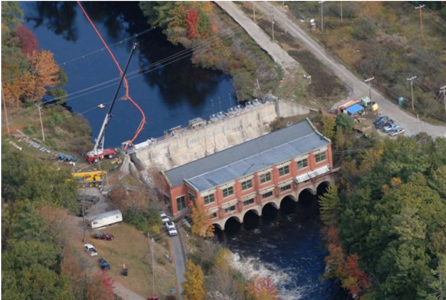
FIGURE 1-4. BONNY EAGLE INTAKE, POWERHOUSE AND TAILRACE - AERIAL
