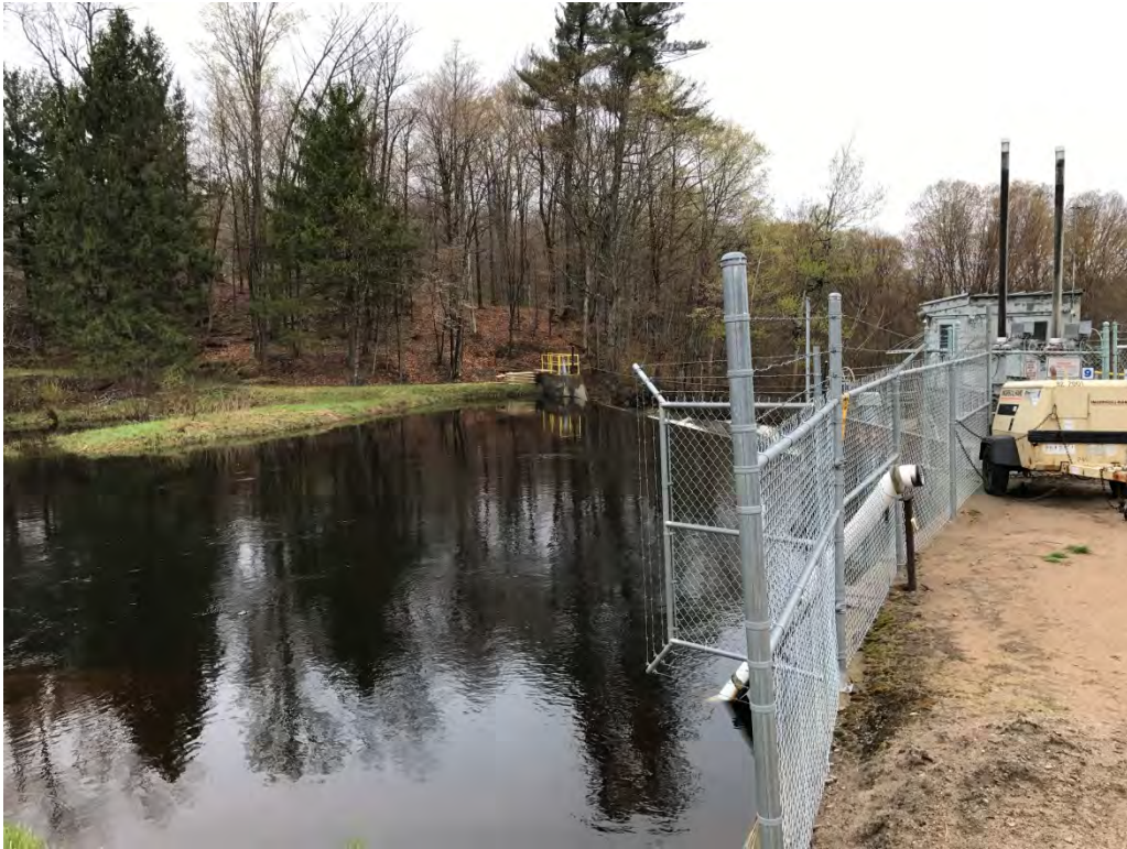
Spillway and intake structure
