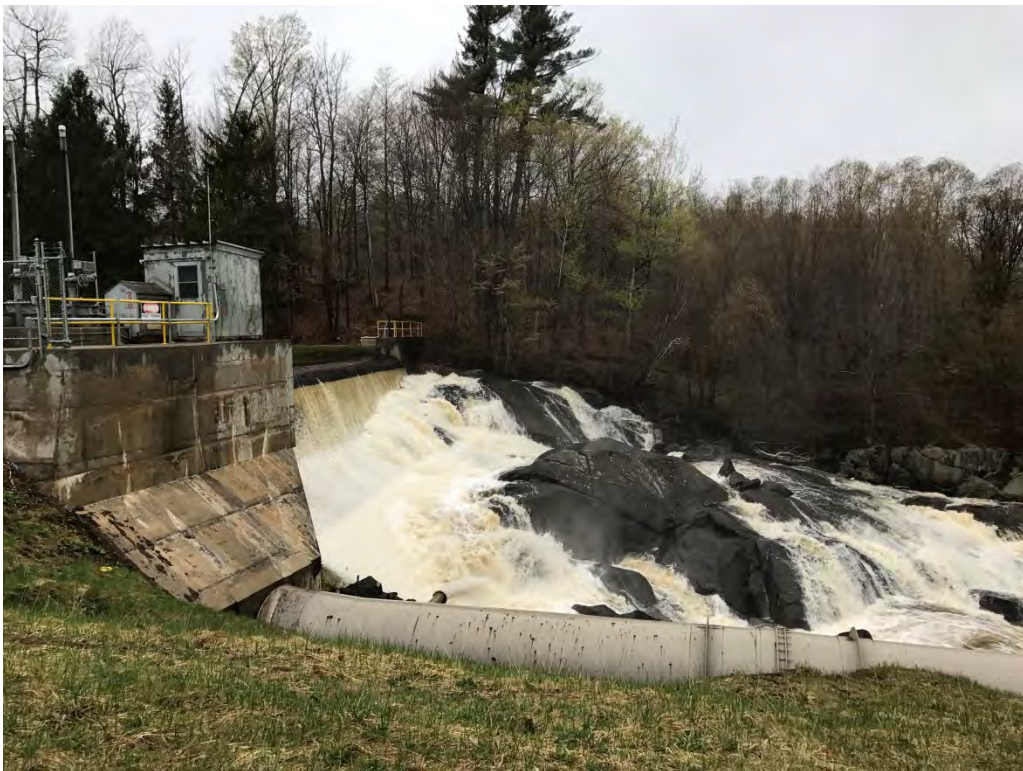
Spillway and intake structure
