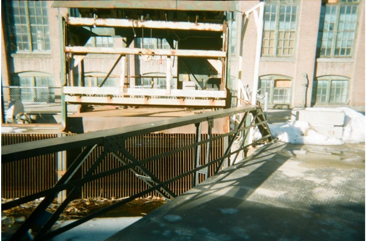
Intake Structure (Includes Forebay, Penstocks & Trackracks)
