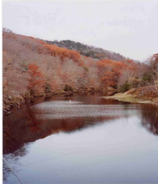
Deerfield No. 5 reservoir, looking upstream from the dam. (LIHI)
