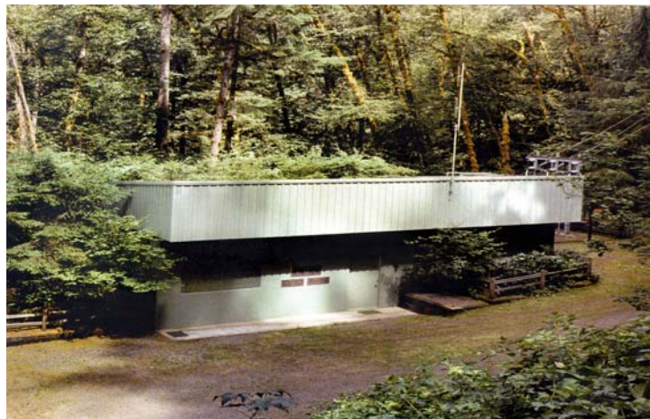
Falls Creek Powerhouse (photo by Frontier Technology, Inc.)
