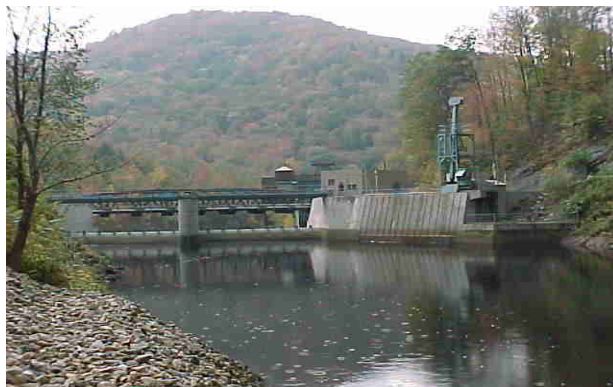
Deerfield No. 5 dam looking at it from upstream (PG&E NEG)
