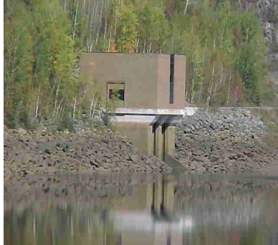
Deerfield No. 5 powerhouse at the Fife Brook Impoundment (PG&E NEG)
