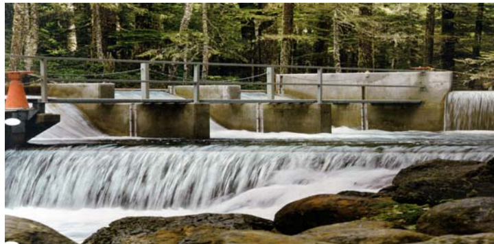
Falls Creek diversion dam (photo by Frontier Technology, Inc.)
