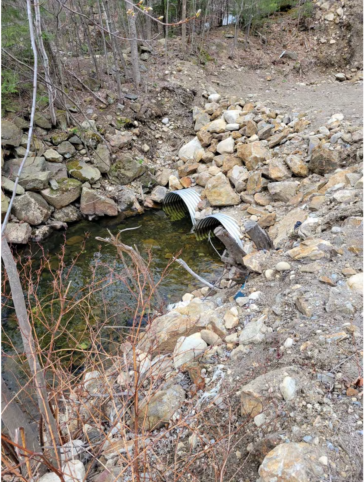
Photo 4 – Repaired Culvert
