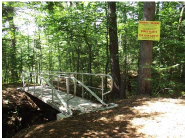
Figure 2 - Newly-constructed pedestrian access
