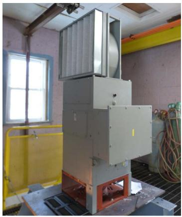
Figure 9. Oemer Permanent Magnet Generator allows variable flow operation
