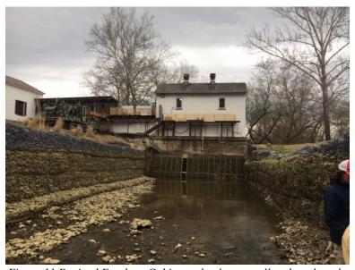
Figure 11 Drained Forebay, Gabion embankment wall and trash racks
