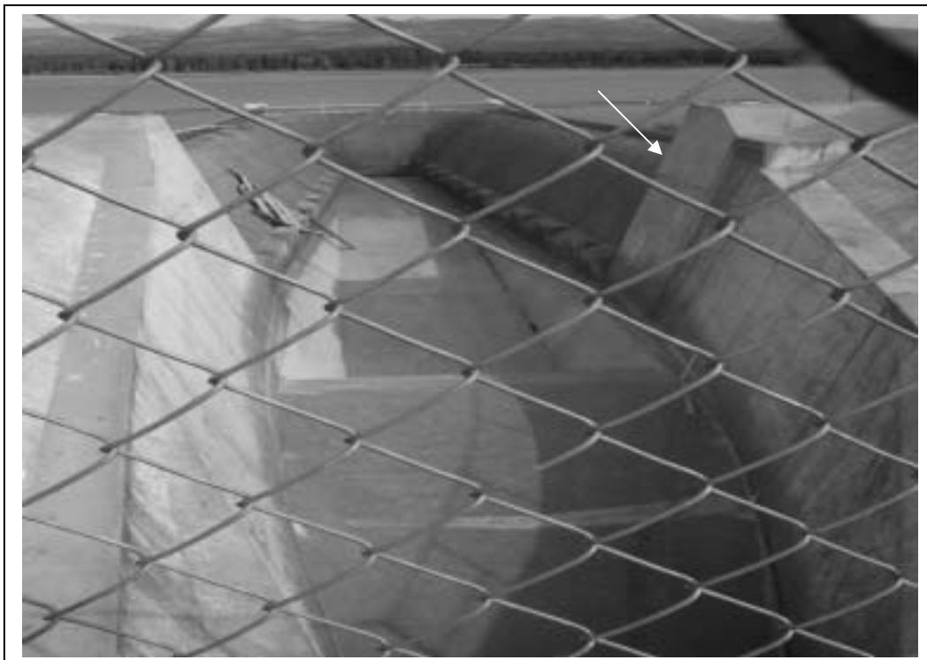
Photo #10: View of the spillway at the dam and the reservoir upstream. The arrow points to the rubber extensions used on the spillway.
