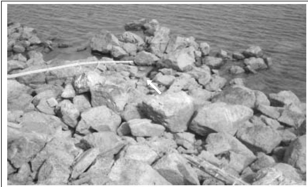
Photo #3: View of cement penstock leading to the intake at the bottom of the reservoir (arrow).
