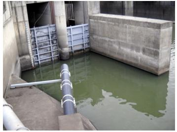
Figure 3. Fish bypass outfall at tailrace entrance to N1 ladderr
