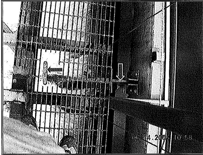
Photograph No. 4 – Stanchion Tripping Mechanism. Pin at Right is Removed Prior to Pulling Handle at Left.
