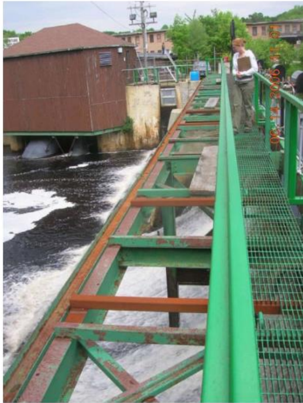
Photograph No. 3 - Walkway over the Dam& Marden Style Needle and Stop log section looking North.
