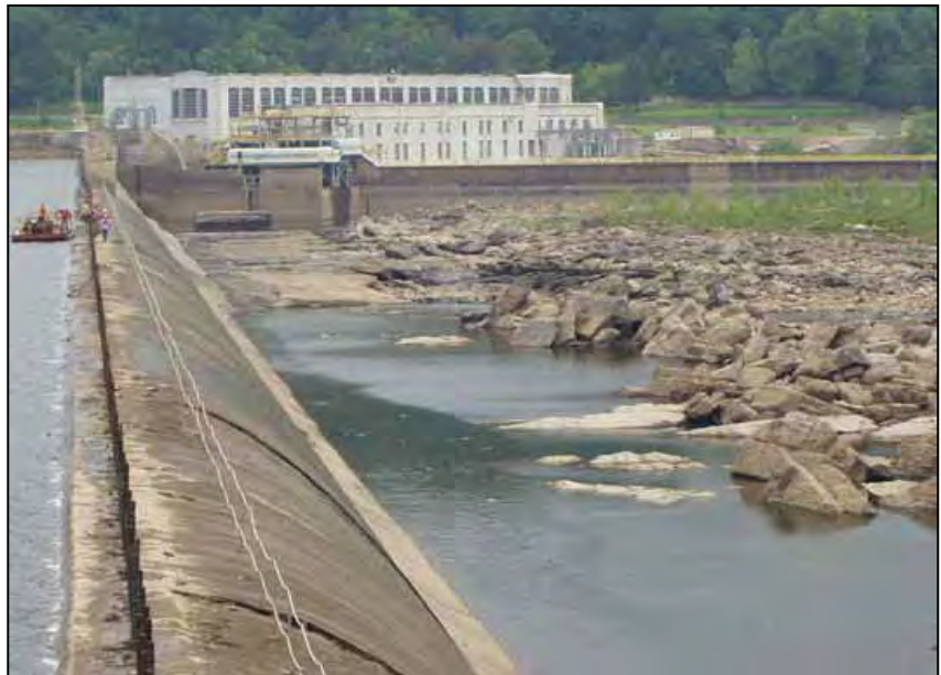
Photo 2 - EXISTING POWERHOUSE AND DAM PRE-REDEVELOPMENT
