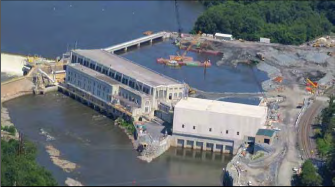
Photo 3 - AERIAL VIEW OF NEW POWERHOUSE CONSTRUCTION ON JUNE 15, 2013
