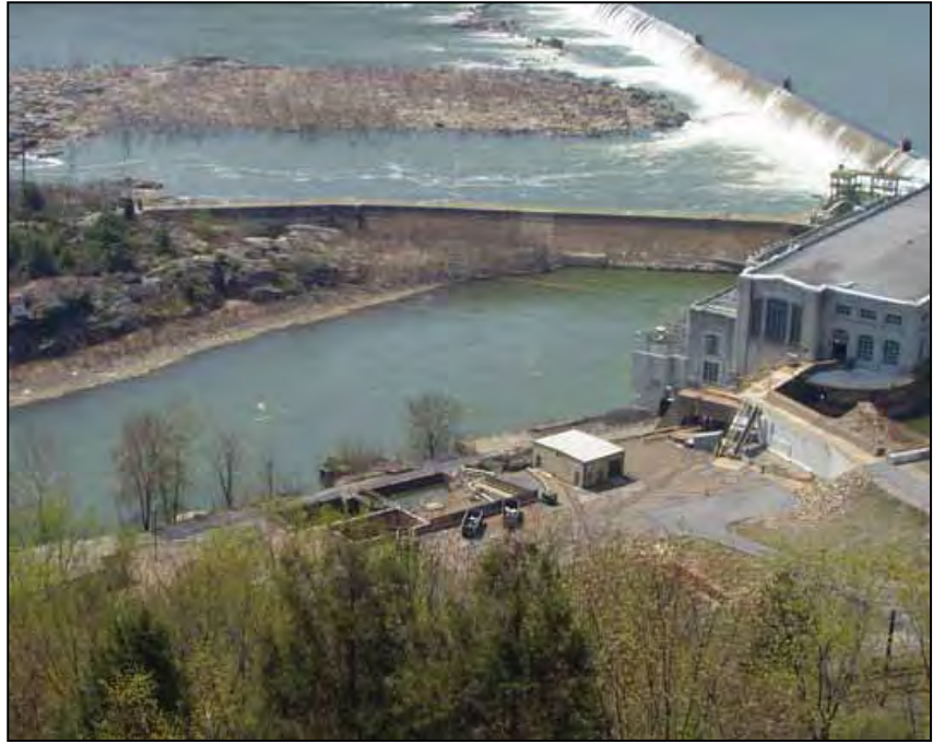
Photo 1 - EXISTING POWERHOUSE PRE-REDEVELOPMENT
