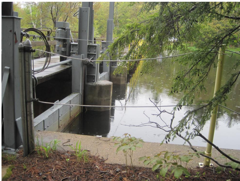
Figure 6. East section of dam from Maine side showing two sluiceways, one of which is adjusted to release the bypass minimum flow.
