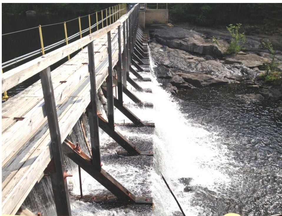
Figure 5. West section of dam looking towards Maine shore. The struts support the stanchion stoplogs.
